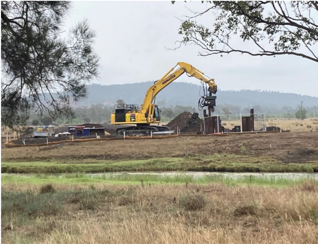
Photograph 5 - Twelve Mile Creek, removal of sheet piles from tunnel boring pit. Note waterway in foreground undisturbed by trenchless crossing method.
