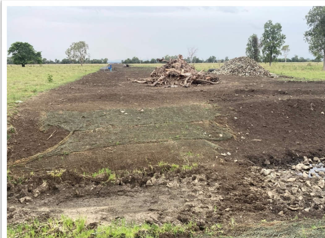
Photograph 2 – CH 35000 (approx.), Waterway crossing with jute matting and hydro mulching to stabilise embankment.
