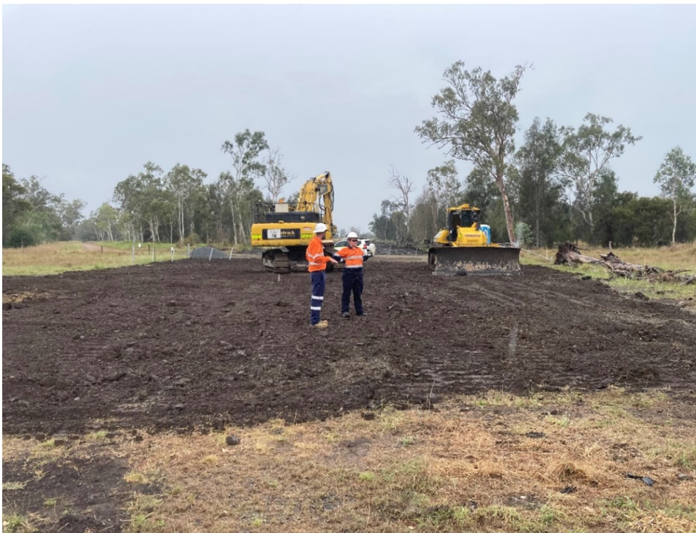
Photograph 6 – CH 37000 (approx.) Pipeline Right of Way reinstalment work underway to replace topsoil and reprofile to match existing levels.
