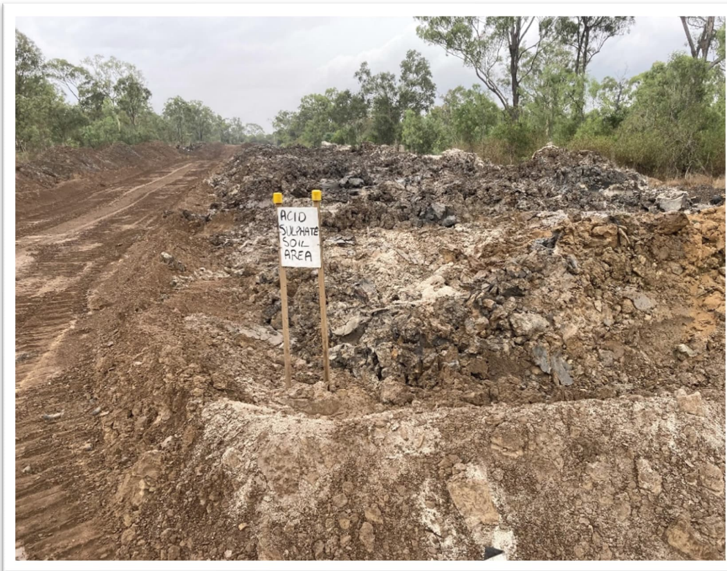
Photograph 7 – Near Raglan Creek, Potential Acid Sulphate Soil temporary bunded stockpile area.
