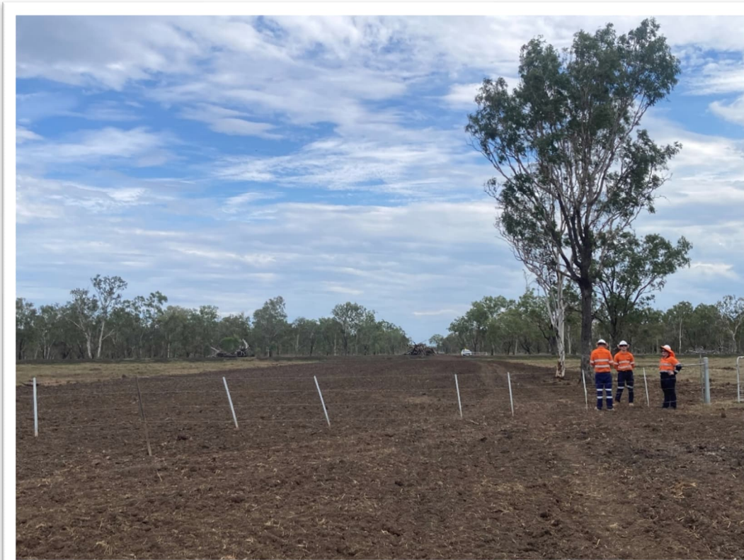
Photograph 1 – CH30000 Pipeline Right of Way topsoil reinstated and reprofiled to match exiting levels.
