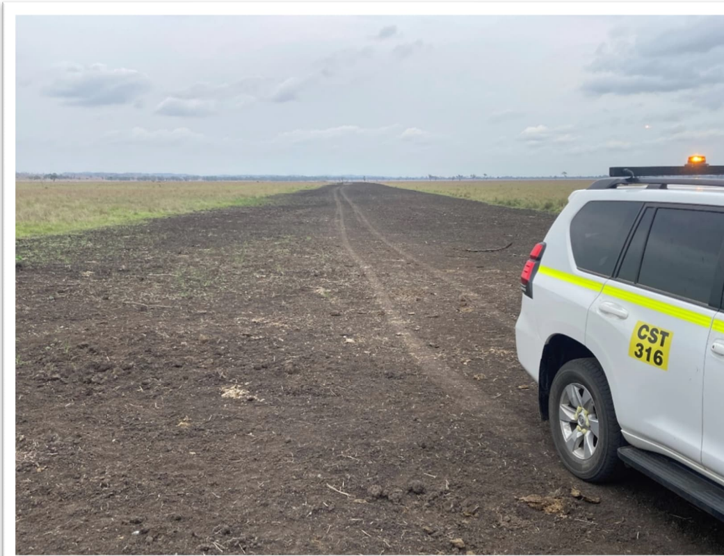
Photograph 3 - Pipeline Right of Way topsoil reinstated and reprofiled to match exiting level, with early regrowth.
